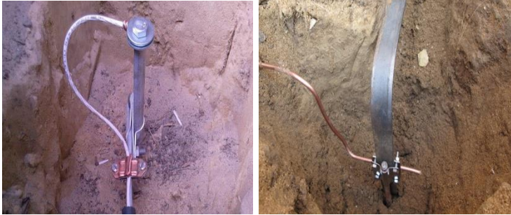
Fig. 5.13. Device trench installation of vertical electrodes
