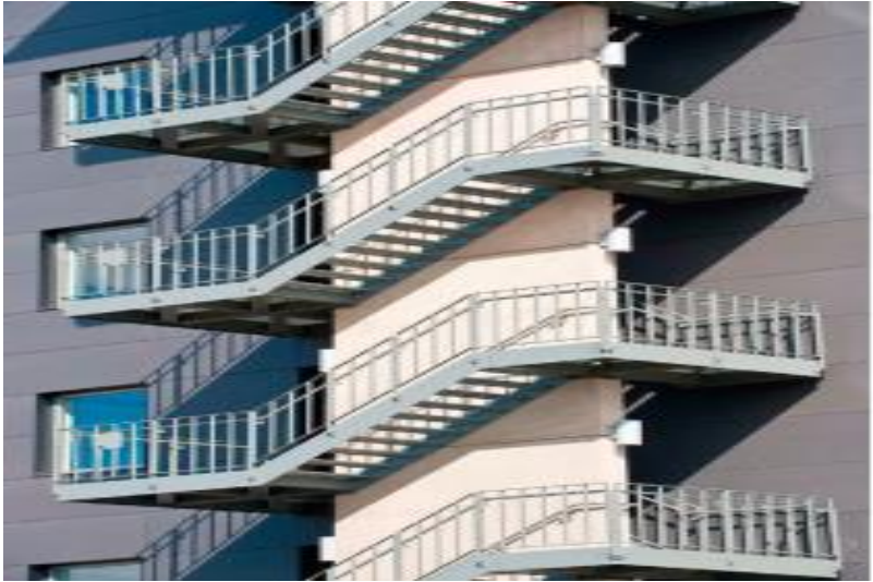
Fig. 10.2. Fire stairs of a multi-storey building
