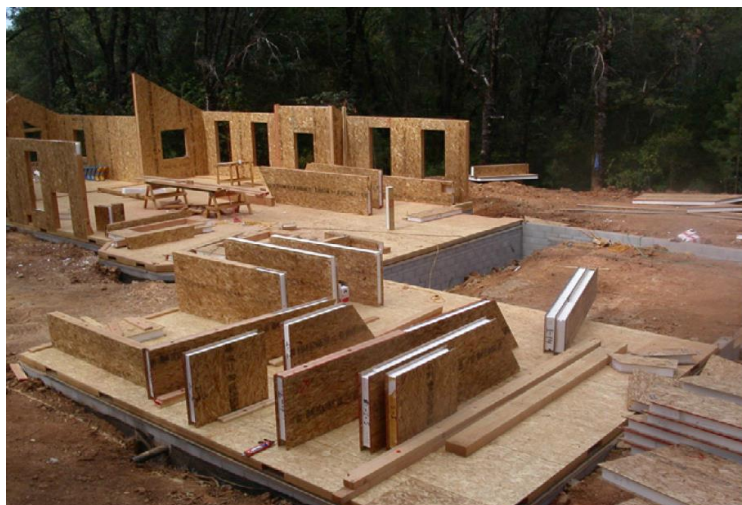
Fig. 10.6. Main insulation panels of buildings
