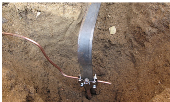
3.9 – rasm. Vertikal elektrodni transheyaga o'rnatish qurilmasi
