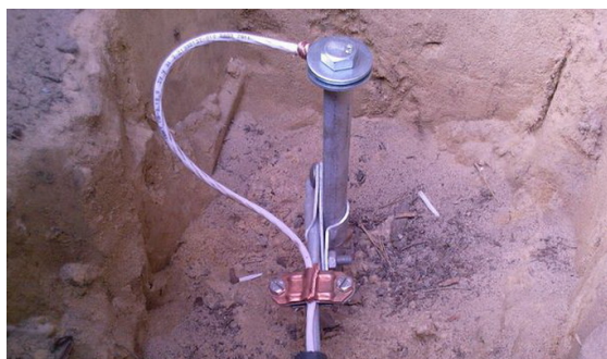
3.9 – rasm. Vertikal elektrodni transheyaga o'rnatish qurilmasi
