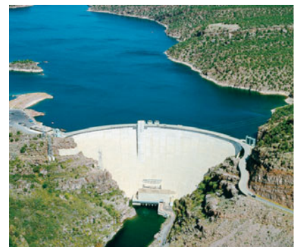
FIGURE 15–27 Problem 55: Flaming Gorge Dam on the Green River in Utah.
