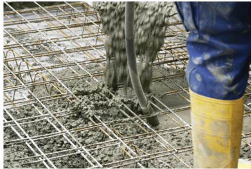
FIGURE 9–26 Steel rods around which concrete is poured for strength.
