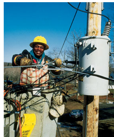
FIGURE 21–22 Repairing a step-down transformer on a utility pole.
