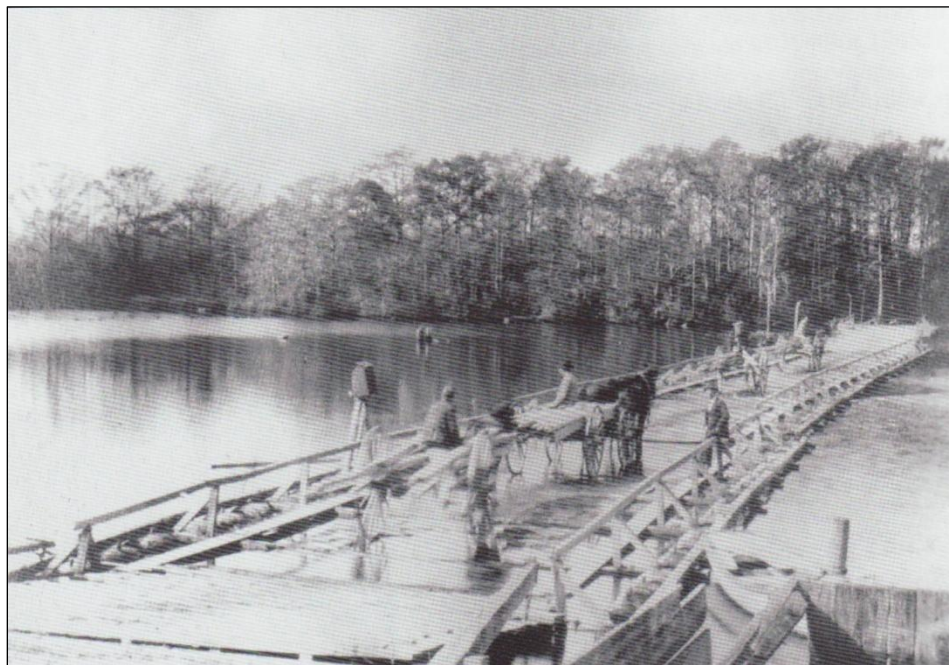
FIGURE 7. Perquimans Float Bridge, c. 1895 (Perquimans County Library 2003:114).
