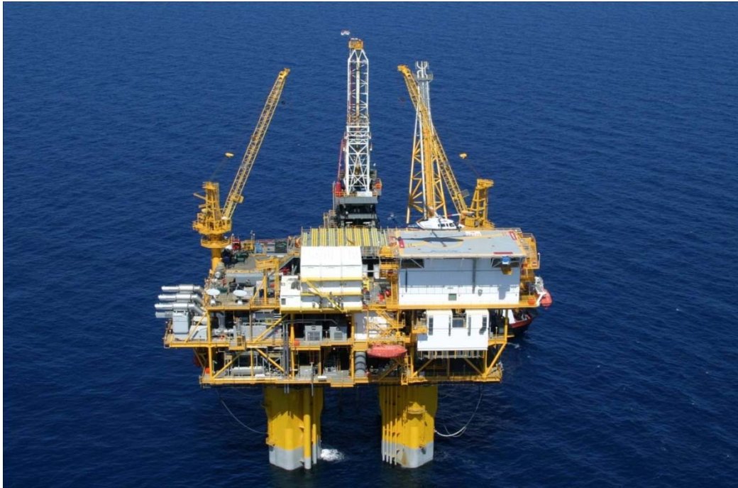
Figure 1: Image of deepwater semi-submersible rig
