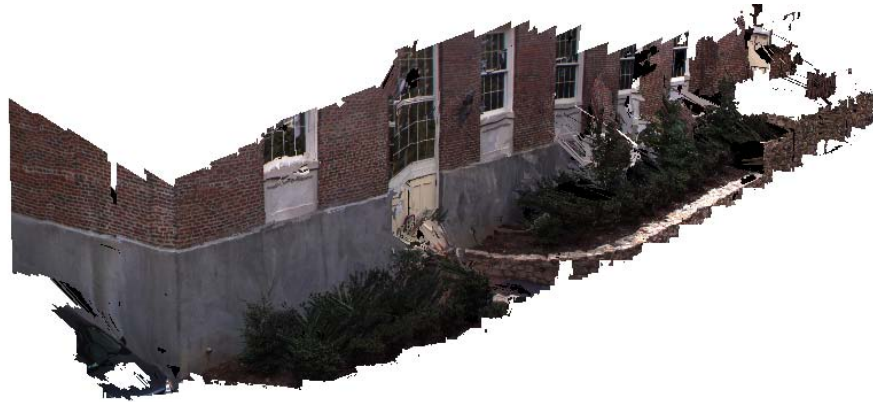
Figure 4.9: The reconstruction produced by our algorithm from several hundred frames of video. By testing only plane hypotheses with high prior probability, the reconstruction was achieved with only 48 plane hypotheses per frame at a speed of 50.0 Hz.
