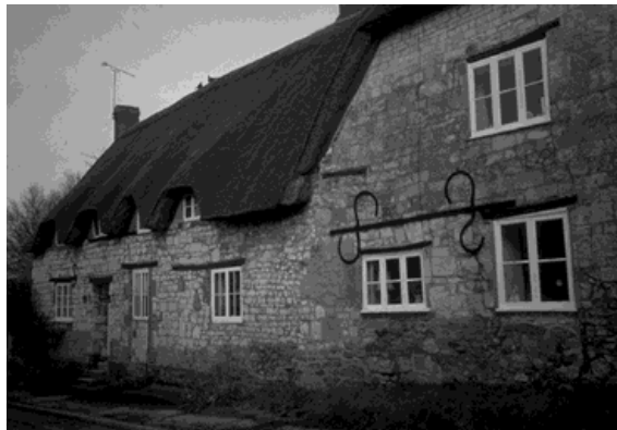
Fig. 3. A sarsen cottage in Oxfordshire, UK.
