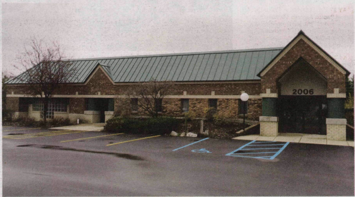
QUANTUM LEAP'S new facility is more than triple the size of its old one. The company will rent space inside the building to clients and nonprofits until it grows large enough to occupy the entire site. Courtesy Quantum Leap
