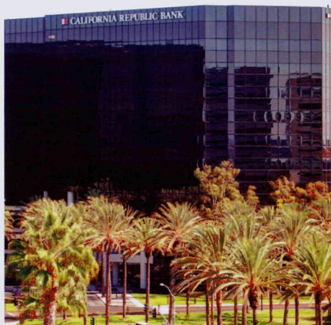
New headquarters: put name on Irvine Towers building after move to accommodate growth
