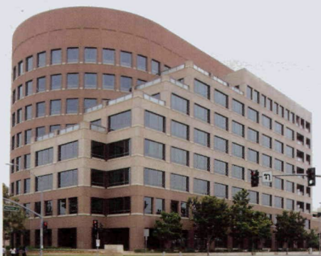
1750 E. 4th: deal calls for transportation agency to buy smaller of the two buildings at Xerox Centre campus in Santa Ana
