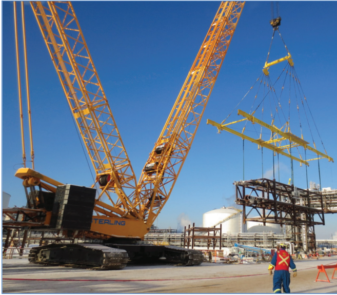
Fig. 1. Module lifting by a mobile crane at an industrial site.
