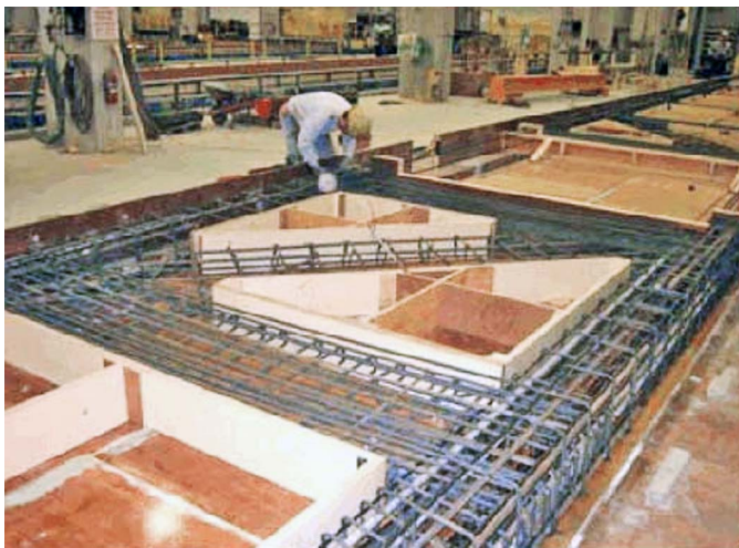
Fig. 5. Precast truss fabrication (photo courtesy of the Spancrete Group, Inc.)
