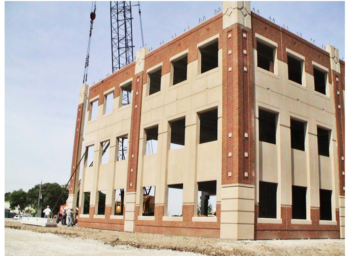
Fig. 3. Precast example: Structure 1 (photo by J. Zachar)
