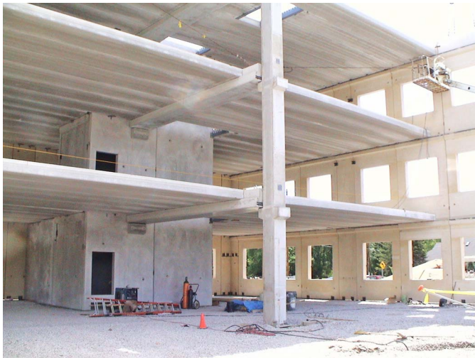
Fig. 4. Precast example: Structure 1, plank beams, and columns (photo by J. Zachar)
