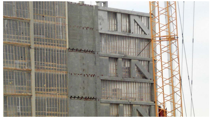
Fig. 6. Precast truss erection (photo by J. Zachar)
