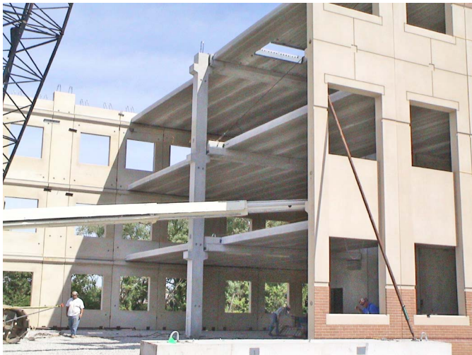
Fig. 2. Precast example: Structure 1 (photo by J. Zachar)
